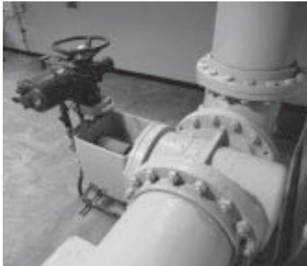
18" Cam-Centric® plug valve with motor actuator.
